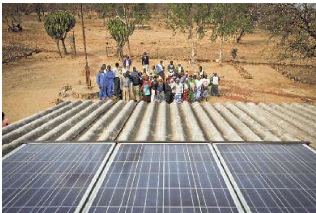
Solar panels provide the clinic in Chitulipasi with electricity.
