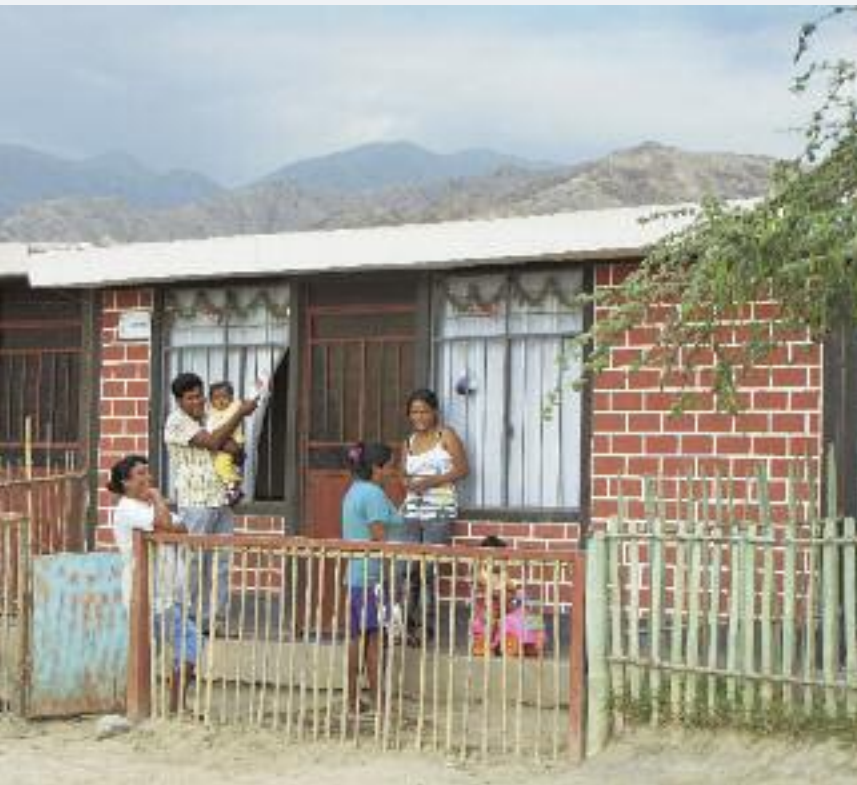
The new houses made of cane and concrete are earthquake resistant.
